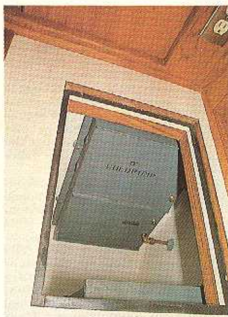
Typical hold-over plate in a freezer marked for 0°F. This indicates a strong salt solution inside the plate. Note pipe entering box is well sealed to cut heat transfer.
